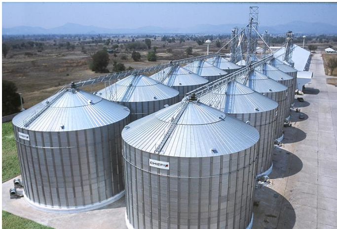
Figure 4: Battery of silos for bulk storage of food grains
