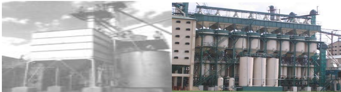
Fig3: Industrial Parboiling system
