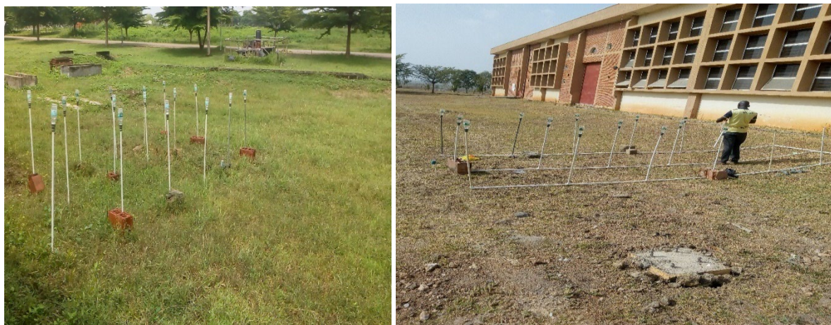
Plate 1- Installation and Settings and Fittings for the Sprinkler Head
