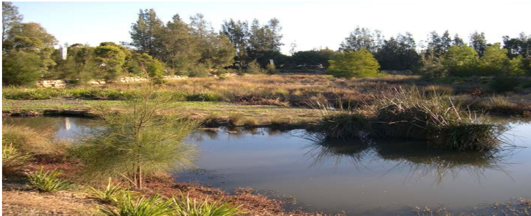
Figure 1: A free water surface constructed wetland (FWS CW) for stormwater runoff
